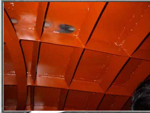
After ( Coated with Acourete Paint EZ1 )
