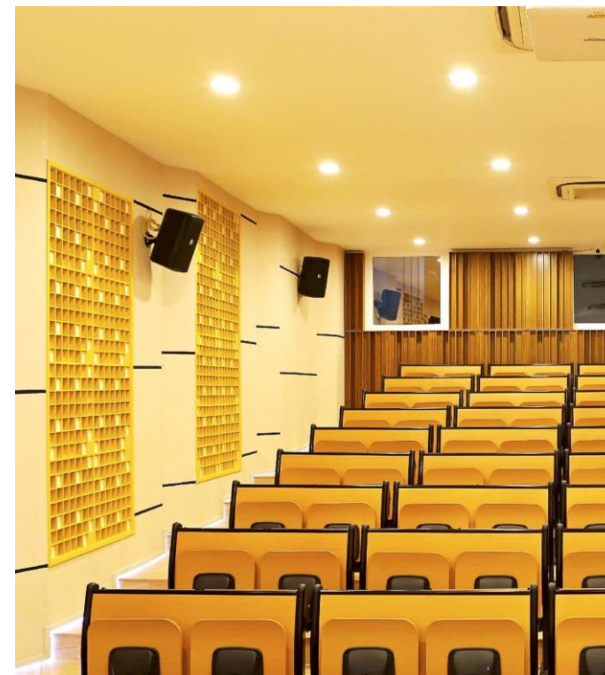
Use acoustic material for additional treatment
