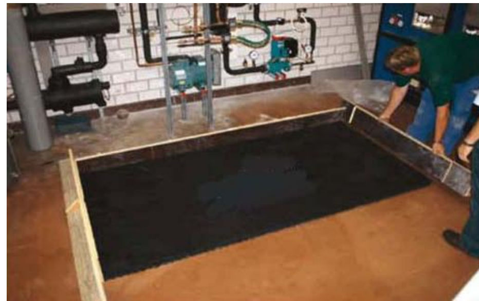
1 tiles or other floor coverings • 2 glue • 3 screed • 4 PE foil • 5 Regupol® or Regufoam® screed insulation • 6 raw ceiling • 7 perimeter insulation strips made of Regupol® , Regufoam® or another material
